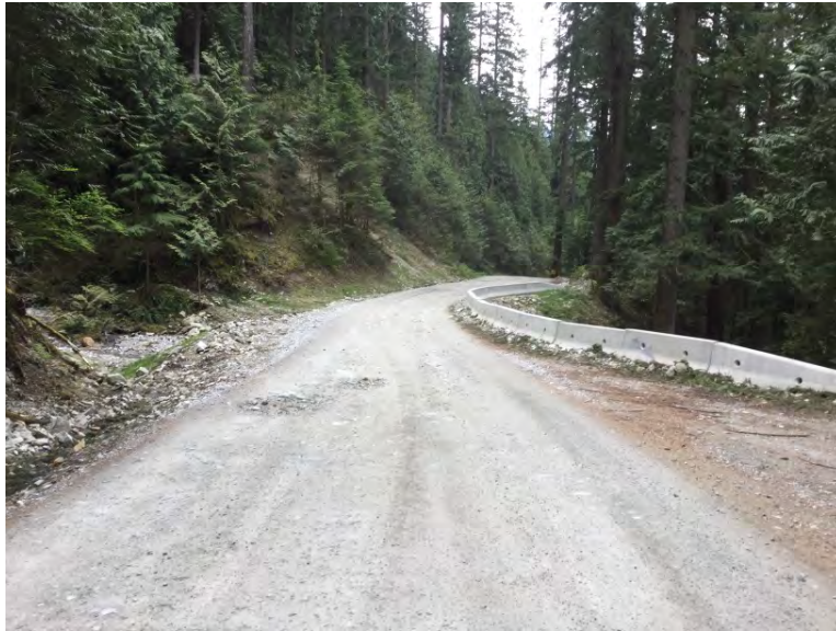
Approach from Right Bank when facing downstream
